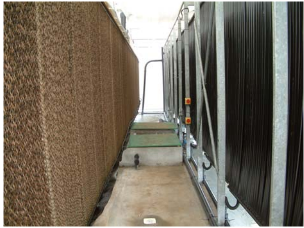
Cardboard evaporator, reinforced by \text{CaCO}_3 bio-mineralisation from seawater, and polythene tube heat exchanger.
