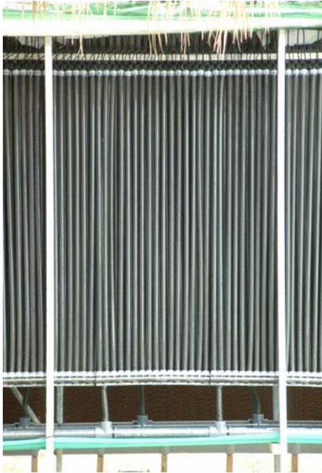
Assembly on site of the 'Watermaker' all plastic condenser.
